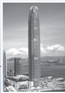
IFC Tower 2 completed
